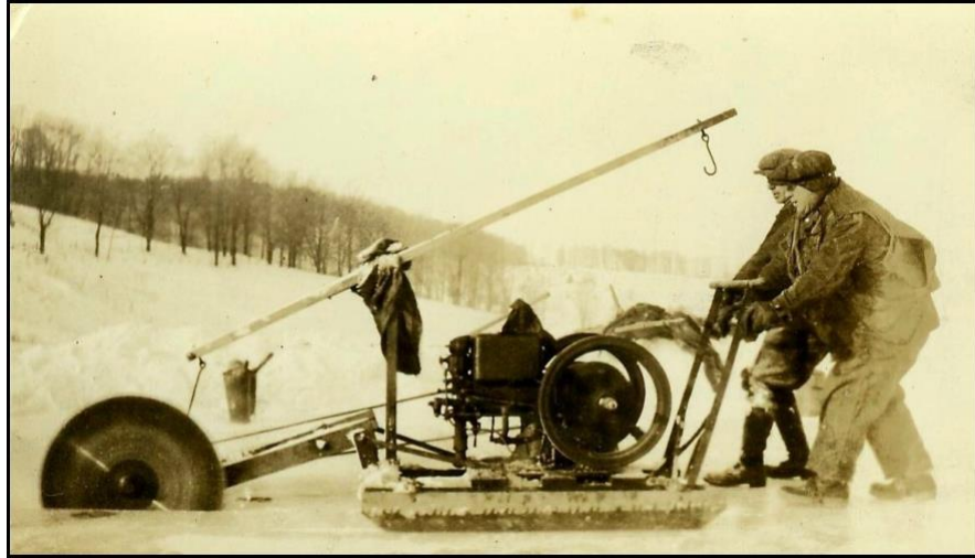
Sawing blocks of ice
